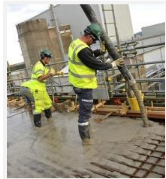
In-situ concrete pouring and formwork
